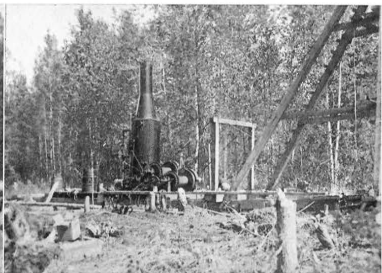
The pile driver at the King River Camp had timber nearby for use
