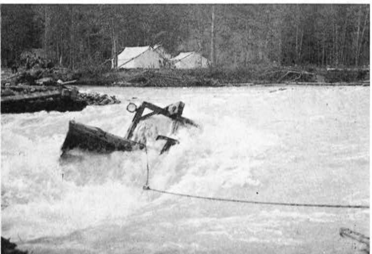
R.D.-8 plunged through a temporary bridge near the King River Camp
