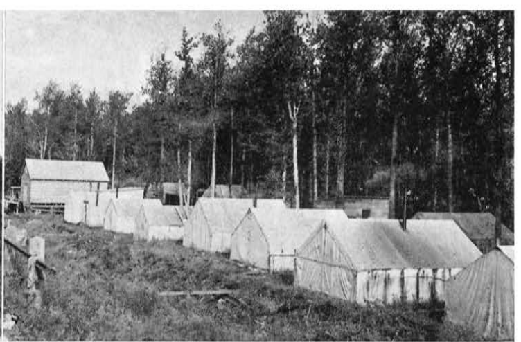
The road construction camp near Sutton was a tented village
