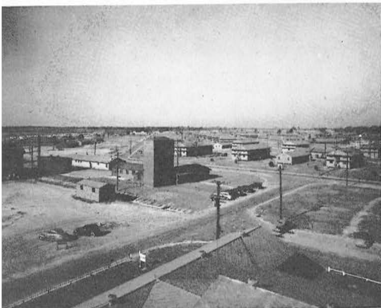
The building of Moody Field, near Valdosta, Georgia, required the moving of one and one-half million yards of earth and included all city installations
