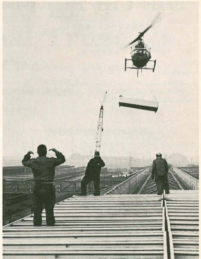
Here comes the "chopper" with 700-pound ventilator ...
