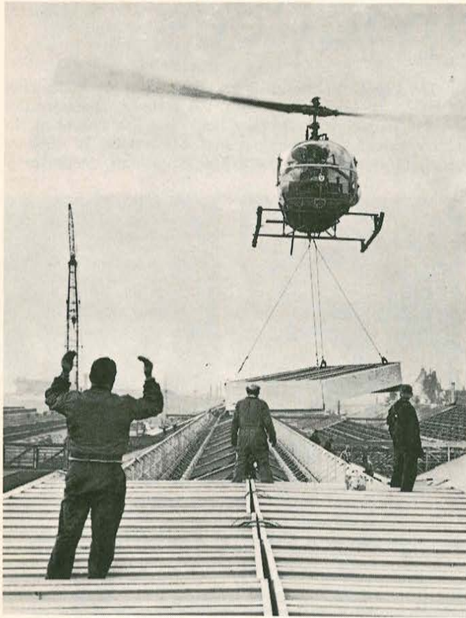
... pilot positions section over spot where it is to rest ..
