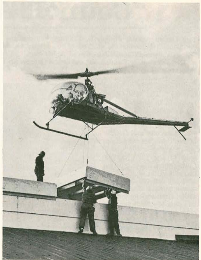
... Outside contractor's men ease the section into place.
