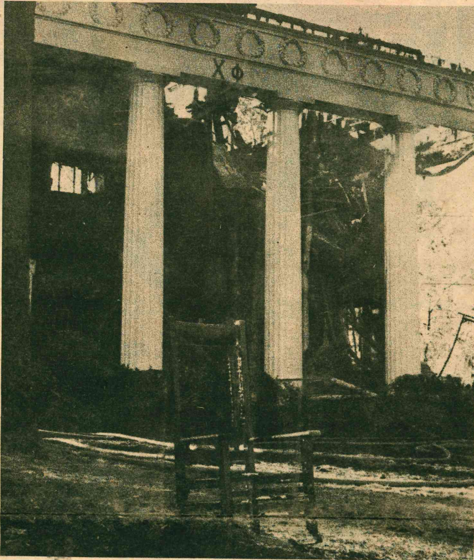
Only the pillars remained after fire destroyed the Gamma House during Christmas holidays a year ago. Rebuilding is beginning.
