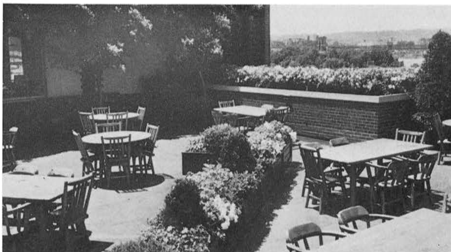
Wiedemann Roof Garden with Cincinnati in background
