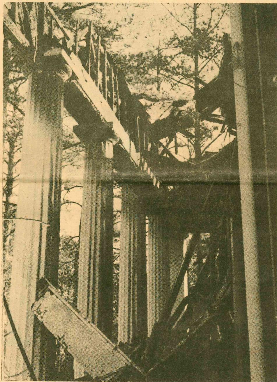
The graceful columns and the kitchen are all that remain of the Gamma chapter house at Eight Fraternity Row on the Emory University campus, following a disastrous fire during the Christmas break (See story on page 3)
